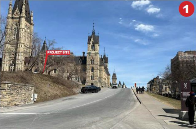
SOUTHWEST: BANK STREET PEDESTRIAN APPROACH
