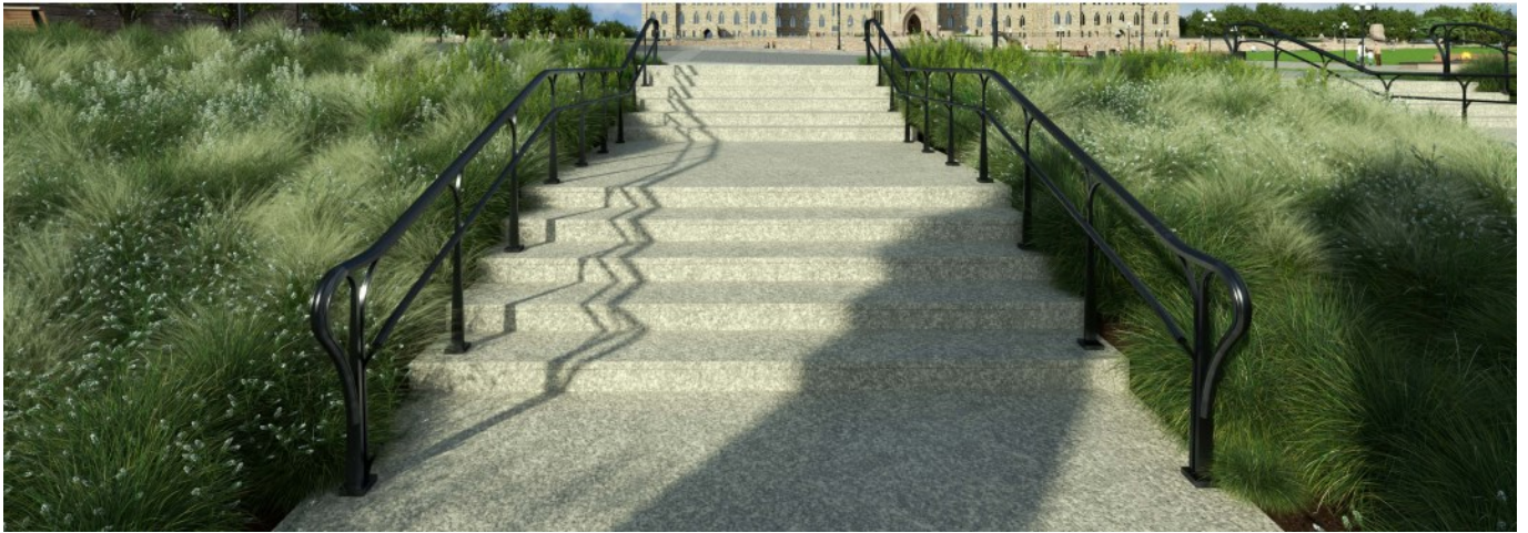
Wellington Street Edge. New stairs entering the Parliamentary Forecourt.
