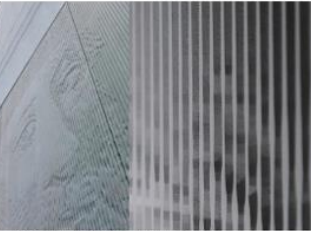
PRECAST CONCRETE PANEL - Photo Engraved
