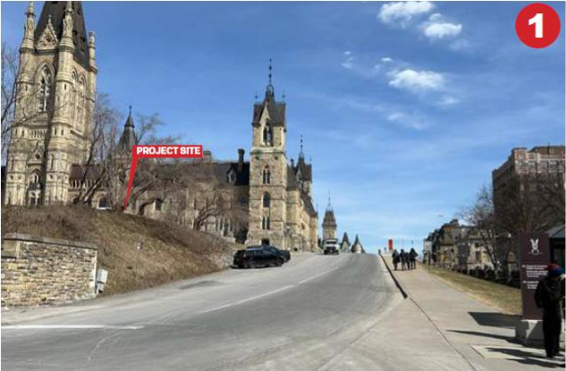
SOUTHWEST: BANK STREET PEDESTRIAN APPROACH
