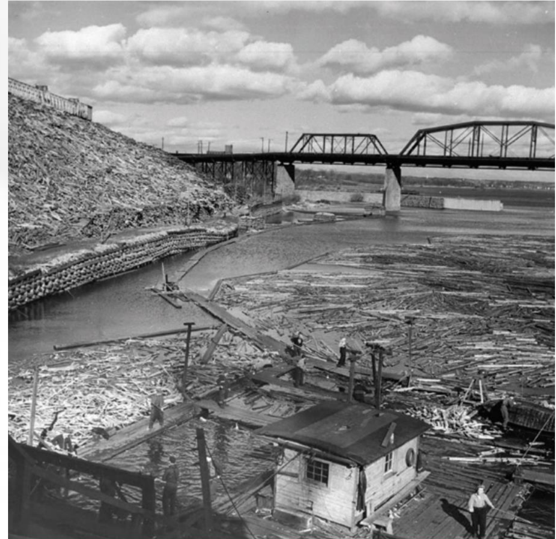
Mountain of logs near the Alexandra Bridge. Canadian Museum of History, 73-534
