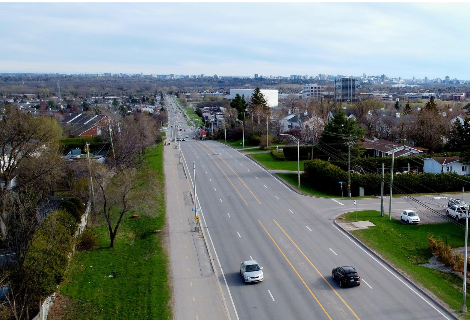
Montée Paiement looking south near rue Lahaie, Gatineau Source: Adham Badran
