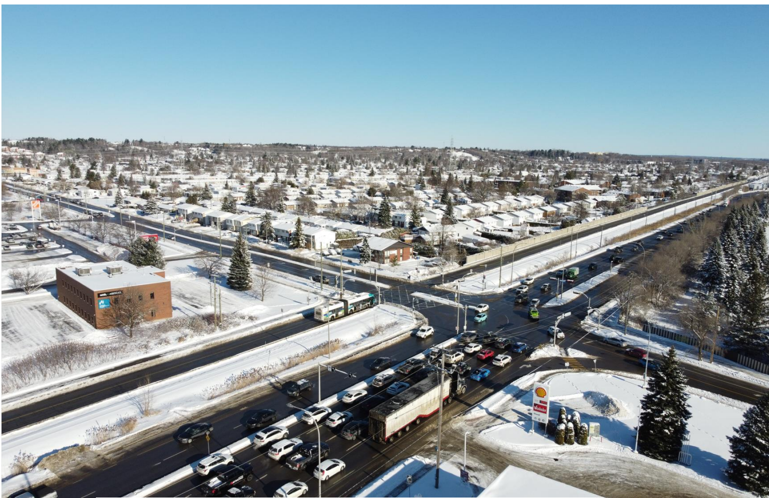
Boulevard Maloney and Montée Paiement intersection Source: Adham Badran
