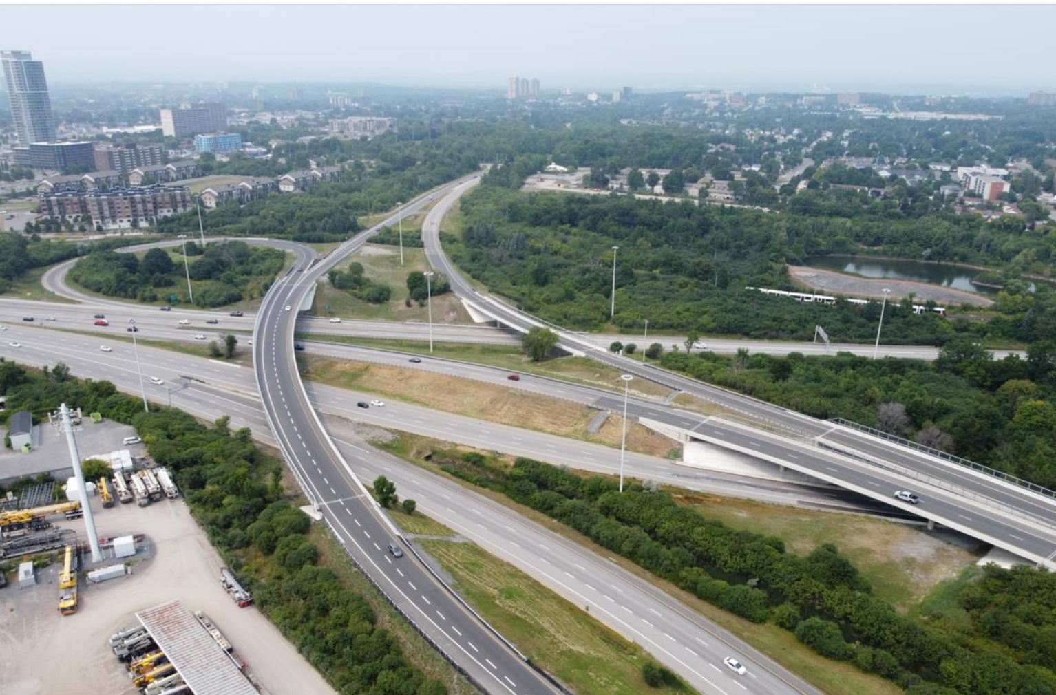
Highway 417 and Ottawa Regional 174 interchange south of Aviation Parkway Source: Adham Badran
