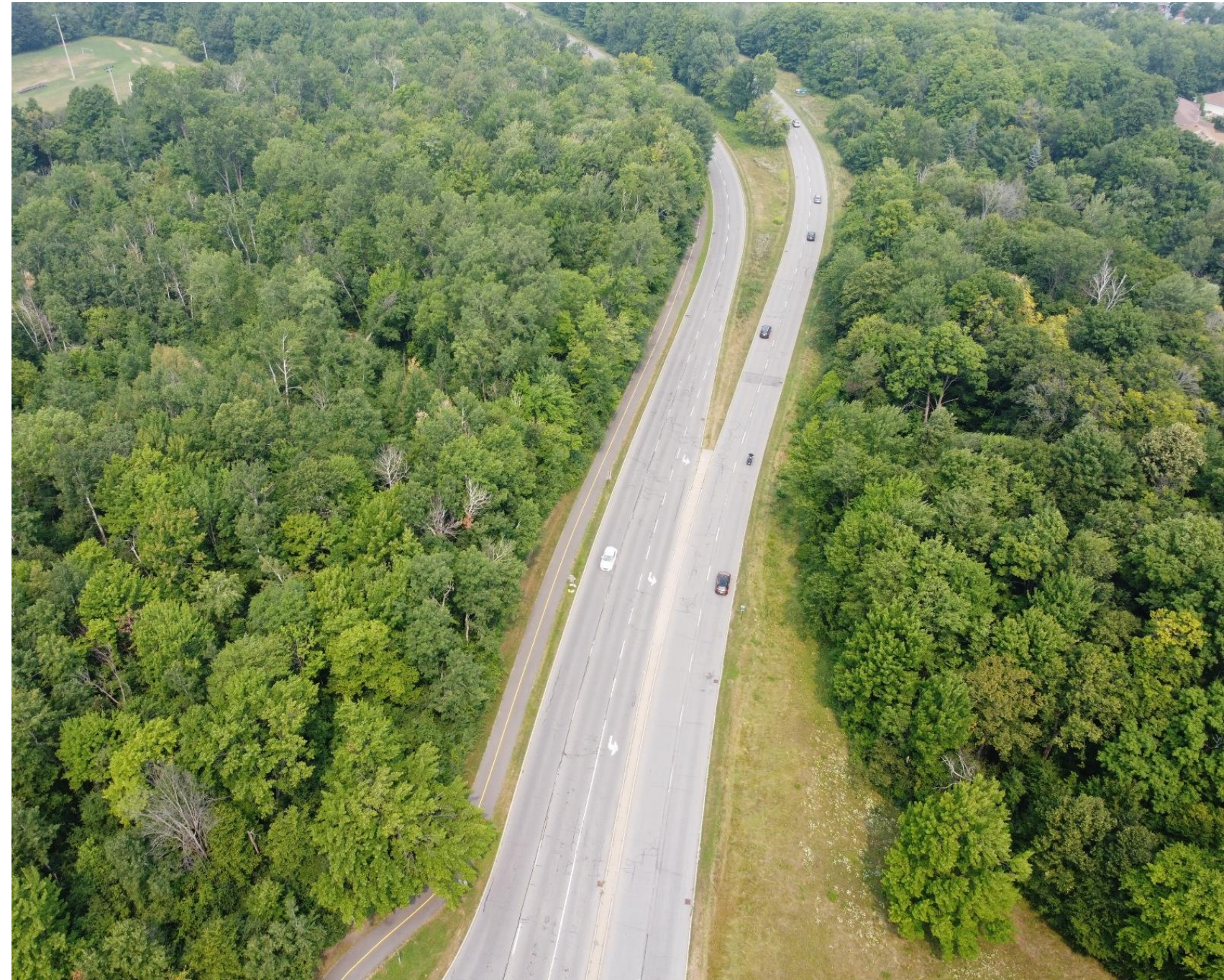
Aviation Parkway looking north from Ogilvie Road, Ottawa Source: Adham Badran
